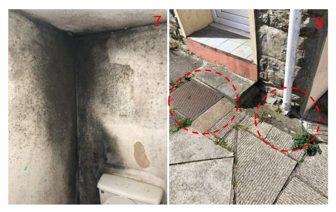
• Picture 8 shows a manhole cover to a drain system and the downpipe that spills onto the street is directly above the damp area in picture 7.
